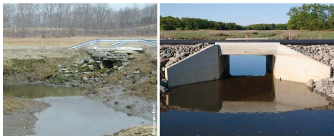
Figure 2 Newman Road culvert crossing replacement (GOMC highlights 2012).
