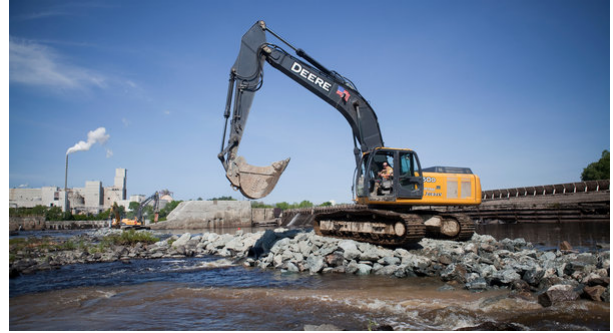
Figure 1 Dam removal process at the Great Works Dam (New York Times 2012).
