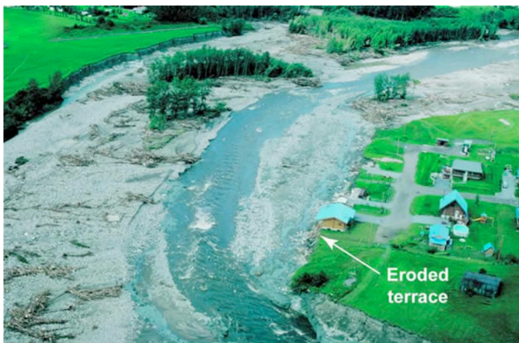
Figure 8: Photograph of buildings on a terrace undermined by bank erosion, Saguenay area, July 1996 (Geological Survey of Canada, photograph GSC 1997-42DD, taken by G.R. Brooks).
