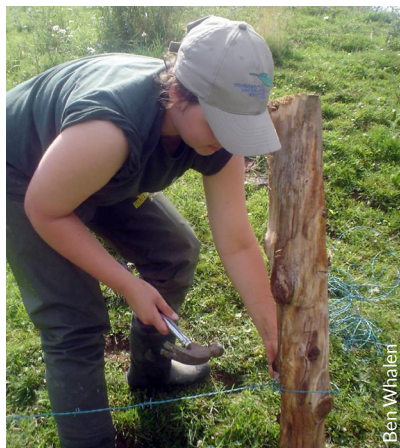
Installation of cattle fencing (left) for restoration of impaired riparian habitat (right).
