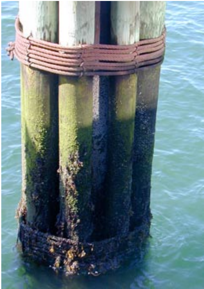
Wooden piling in Boston Harbor, Massachusetts, colonized by a fouling community. Ben Fertig
