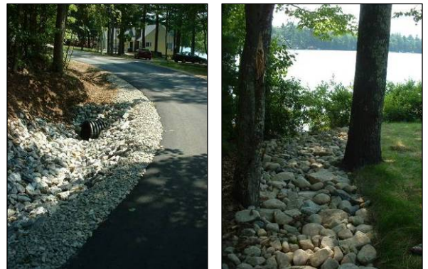
Courtney Lane After – A sediment basin was installed at the top of the road to detain runoff from the adjacent town road. The road was paved, crowned and ditched. The downhill property was stabilized and its buffer was extended.
