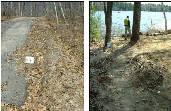
Courtney Lane Before – Severe erosion along the road carried an estimated 20.5 tons of sediment per year across an adjacent property and into the lake.
