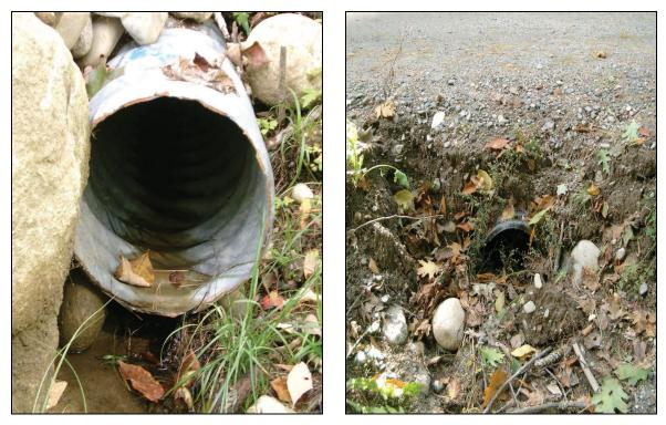
Figures 11 and 12. The picture on the left is a representation of a good culvert with proper drainage and depository pool taken during the road problem survey on 19-Sep-06. The picture on the right is a representation of a poorly maintained culvert as it is filled with debris, has no room for runoff, and no collection pool observed during the road problem survey on 19-Sep-06.
