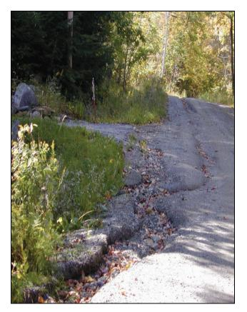
Figure 13. A diversion of some type and a ditch to carry water away from the road are needed to stop the erosion that has already occurred in the image taken during the road problem survey on 19-Sep-06.
