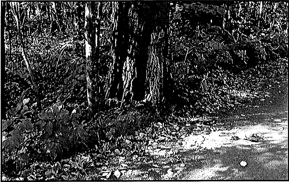
Figure 56. This photograph illustrates a typical berm that can result when grading or snowplowing in the winter causes sediments to build up along the edge of the road, preventing water from flowing off the roadbed.
