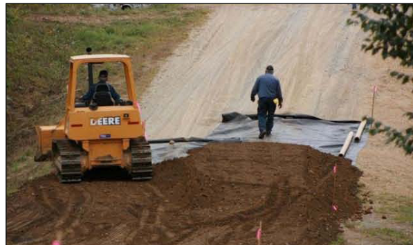
Tarybelu Lane – construction in progress
