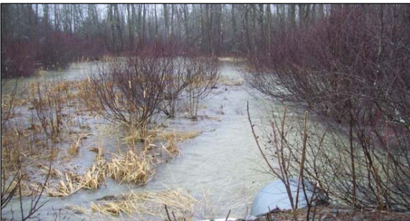
Tarybelu Lane – before construction, silt eroded from road and into lake tributary
