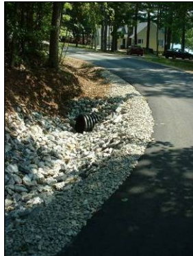
Courtney Lane After – A sediment basin was installed at the top of the road to detain runoff from the adjacent town road. The road was paved, crowned and ditched. The downhill property was stabilized and its buffer was extended.
