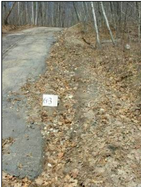
Courtney Lane Before – Severe erosion along the road carried an estimated 20.5 tons of sediment per year across an adjacent property and into the lake.
