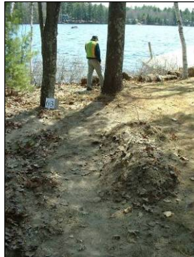
Courtney Lane Before – Severe erosion along the road carried an estimated 20.5 tons of sediment per year across an adjacent property and into the lake.
