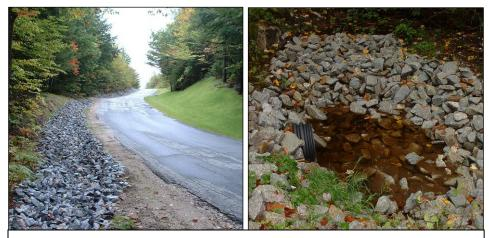
The project addressed three high impact sites on Hardscrabble Road in the Town of Sweden. Work included 850 feet of ditch stabilization, slope stabilization and installation of several turnouts and plunge pools, resulting in a pollutant load reduction of an estimated 20.15 tons of sediment per year.
