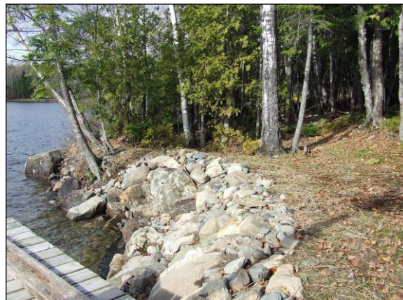
After – Shoreline stabilized with riprap
