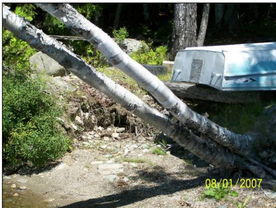
Before - Unstable/eroding shoreline
