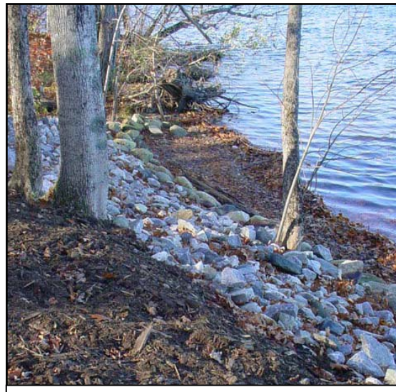
After - Shoreline stabilized with geotextile fabric, rip-rap and Erosion Control Mix
