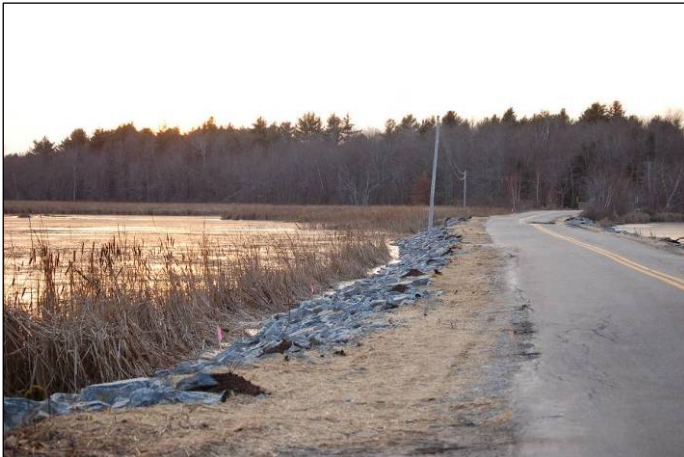
Stabilization of eroding causeway banks
