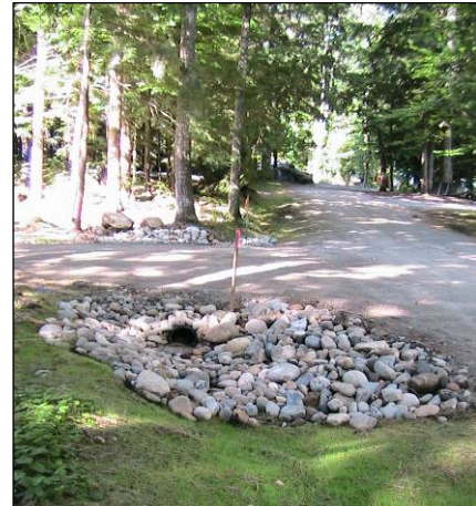
Culvert stabilization project
