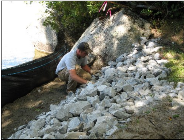
Final touches on a shoreline stabilization project.
