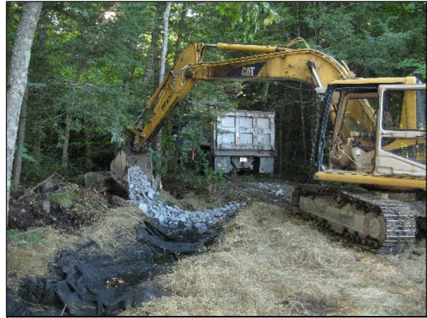
Installation of riprap-lined ditch and plunge pool
