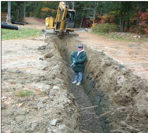
Digging a trench for a new culvert installation.
