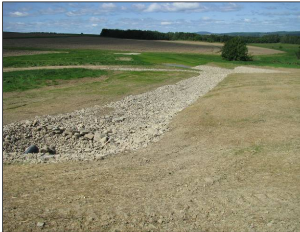
Rock-lined waterways collect runoff from fields
