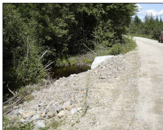
Riprap was used to stabilize sideslopes at the Sinclair Brook crossing on the 45000 road.
