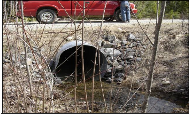
"Squash culvert" that has been installed to maintain stream integrity
