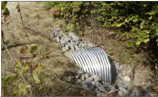
Stabilized underdrain culvert
