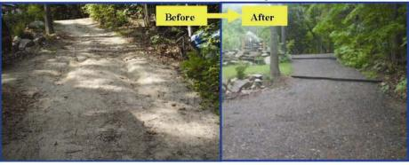
BEFORE: Runoff from Swan's Road (gravel) washes down driveway into the lake. Severe erosion on driveway surface
