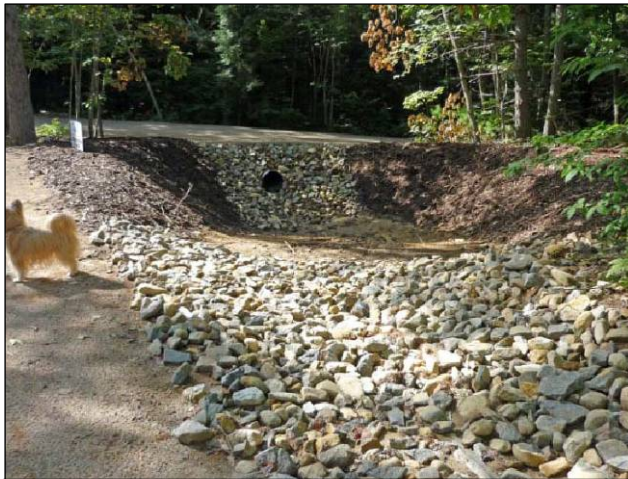
Starboard Lane – This private road was regraded and stabilized, and ditches were installed to carry runoff into this detention basin and then a level spreader.
