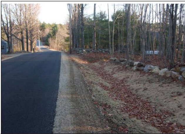
Knox Road – This town road was regraded and paved. Ditches, which were installed on both sides of the road, direct runoff into vegetation and a new detention basin at base of hill.
