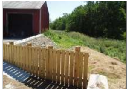
Silage Bunker Vegetated Filter
