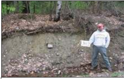
Road survey erosion site
