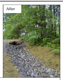
A partially crushed culvert had caused a large washout on this private road. The culvert was replaced; the road and ditch were reshaped and stabilized; and a level spreader was installed at the end of the ditch to disperse flow into the buffer.
