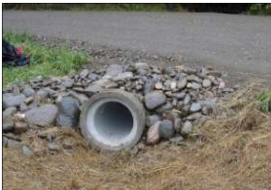
One of many cross drain culverts installed on Bear Lane as part of a road stabilization project
