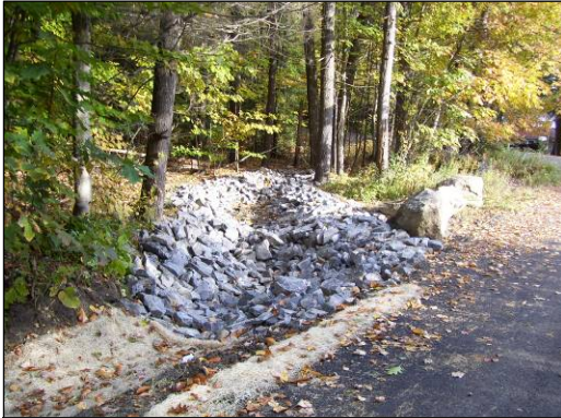
Haven Road – road stabilization, ditching and turnouts into buffers
