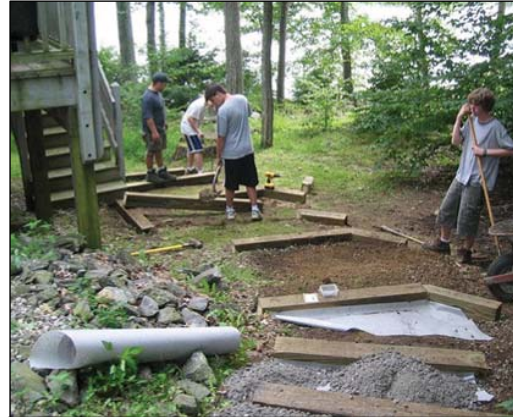
YCC installs infiltration steps
