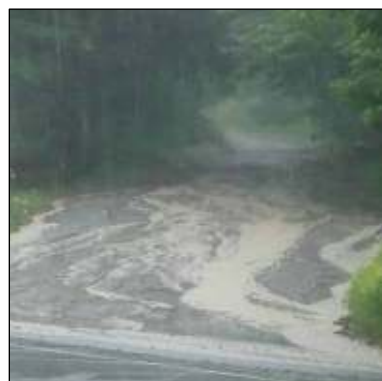
Before implementation, stormwater flowed down Old Cove Road and washed sediment into Cove Brook
