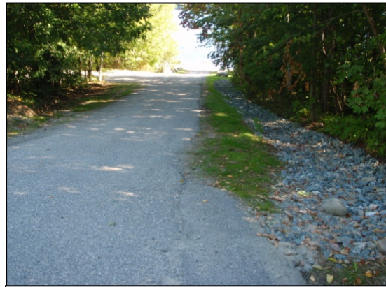
Nicolin Road boat launch after stabilization
