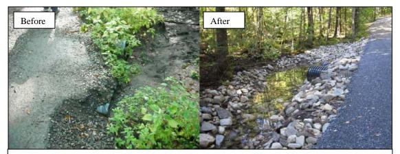
NPS pollution loading from the above road to Long Pond was reduced by replacing a crushed and undersized culvert; armoring the ditch and outlet; and rebuilding the road segment with geotextile, base gravel and crushed bluestone.
