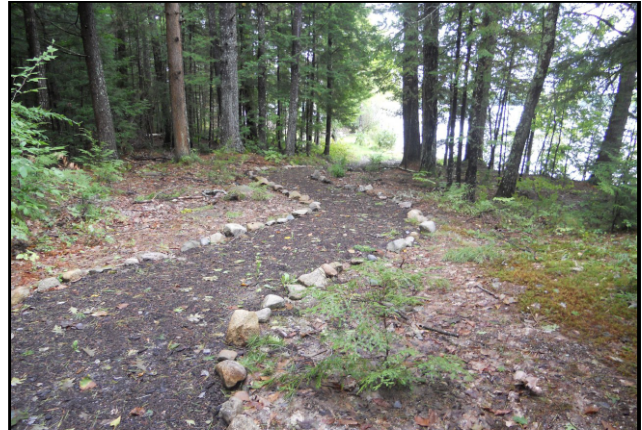
Camp Arcadia installed a meandering pathway down to the lake. Erosion control mulch stabilized the previously eroded path, and stones and native plants helped direct foot traffic.
