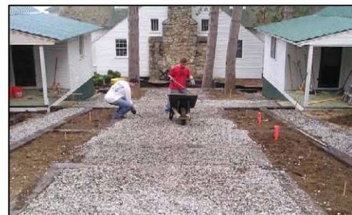
Volunteers stabilized paths, planted vegetation, and installed infiltration steps at Camp O-At-Ka.
