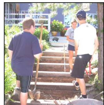
YCC installs infiltration steps at a lakefront property.
