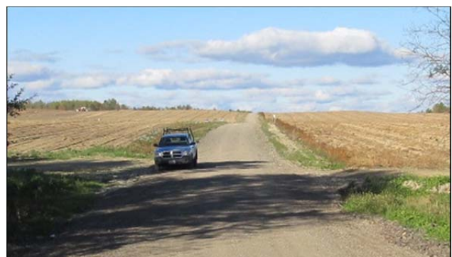
Town road with a grass-stabilized ditch
