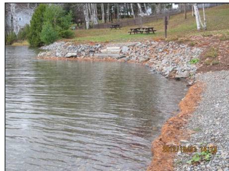
Nickerson Lake shoreline after BMP installation
