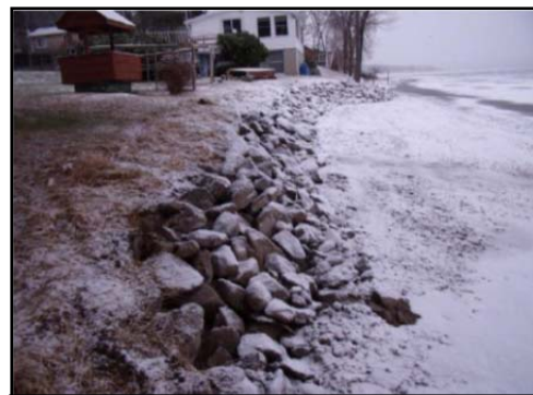
Shoreline stabilization project
