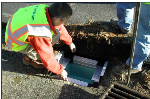
One of 12 filtration BMP catch basin inserts installed on Highland Avenue to trap phosphorus & other pollutants.
