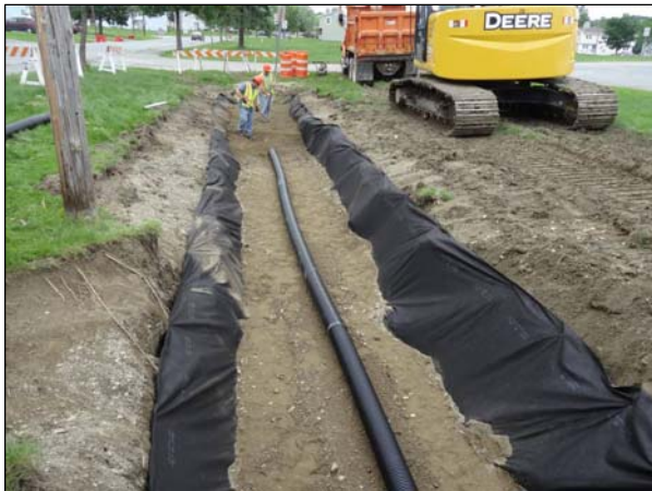
Downeast School biocell during construction.
