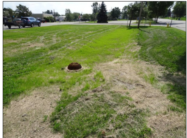
Downeast School biocell after construction.
