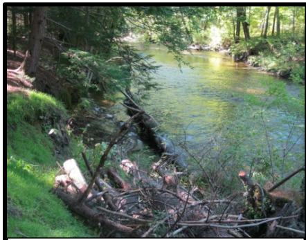
Windham High School trail riverbank stabilization
