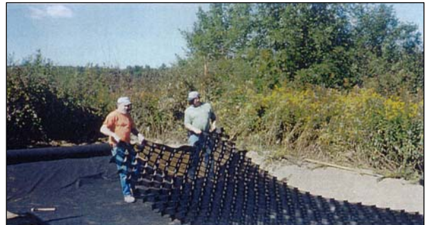
During - Geoweb installation on parking area
