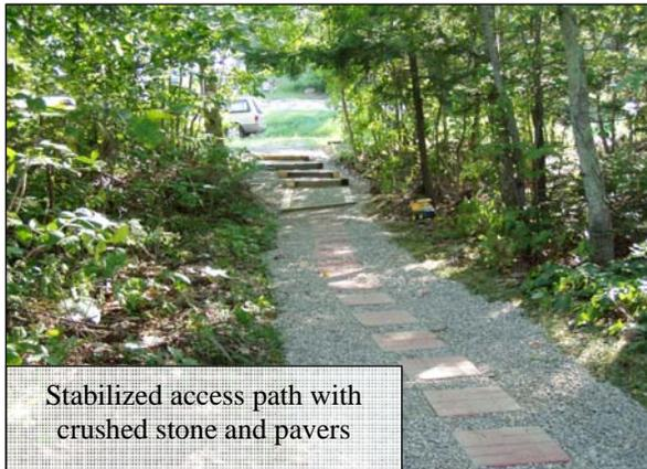
Stabilized access path with crushed stone and pavers
