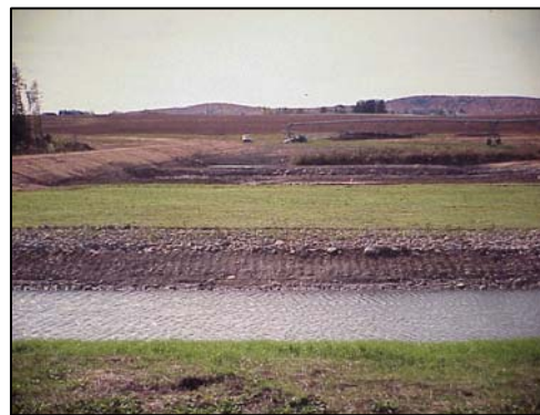
Nutrient & sediment control structure under construction.
