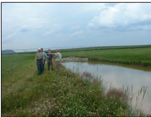
NRCS staff explain how the nutrient & sediment control structure works at BMP tour. (First component of system the sediment basin )
