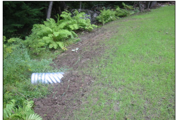
After – Culvert extended. Culvert outlet and road shoulder stabilized.
