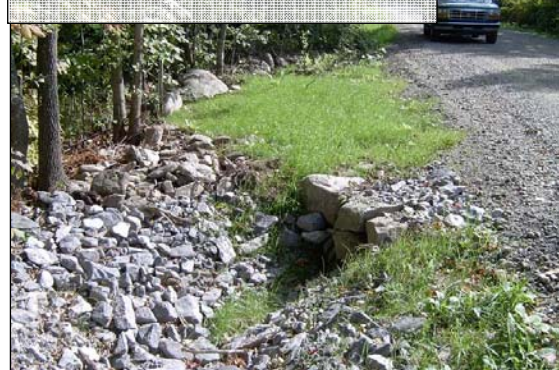
Road, ditch and culvert stabilization
