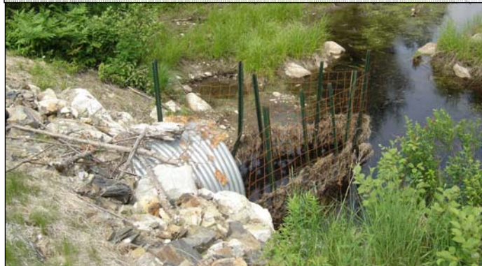
New culvert installed and stabilized with grass and stone. 'Beaver deceiver' installed to prevent new dam construction.
