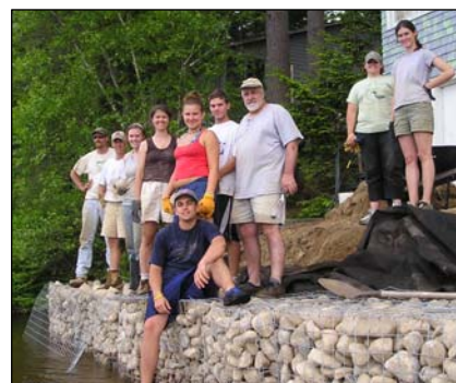
Volunteers install gabion baskets to replace failed retaining wall.
