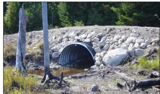
Arch culvert installed to stabilize stream crossing and improve fish passage.
