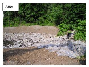
Existing stormwater BMPs at the Rite Aid in downtown Gorham were undersized and unable to handle the runoff. A large rock-lined sediment basin, ditch and checkdams were installed to slow and treat the stormwater.
