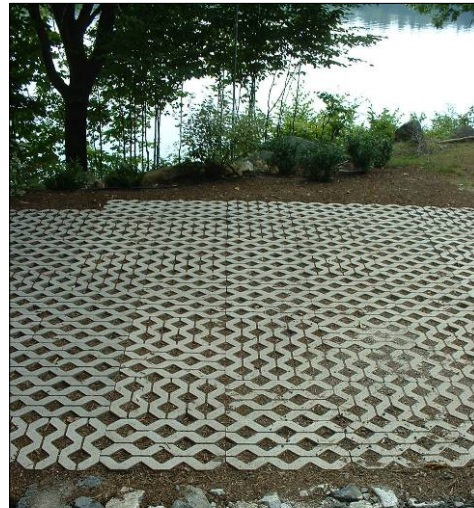
Severe erosion on this steep driveway was remedied by resurfacing with reclaimed asphalt, installing porous pavers on the parking area and planting a buffer next to the lake.
