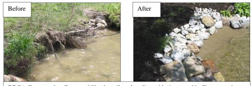
BRCA Conservation Corps stabilized eroding shoreline with riprap and buffer vegetation
