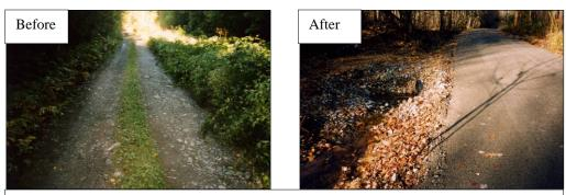
Loon Nest Estates Road – Prior to construction, runoff was trapped on road, which led to erosion of the road surface. Project resurfaced and shaped road and installed ditches.
