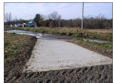
The Veazland Farms project was funded by EQIP and 319. The concrete-lined basin traps solids in the farm runoff, and the liquids are filtered through a vegetative buffer.
