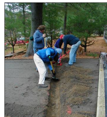
Volunteers build and install waterbars to divert runoff away from lake.
